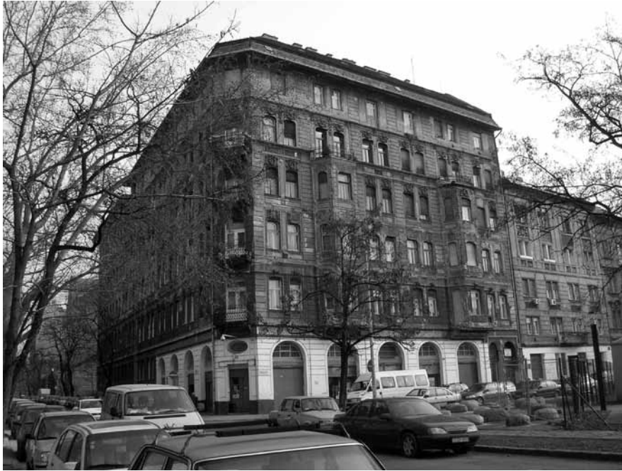
Budapest, Building in rehabilitation. Photo : D.R.
